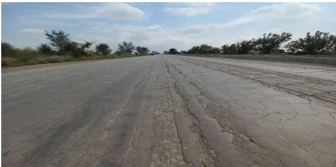
Fig 1. N55 Road Segment near Pezo Bypass
