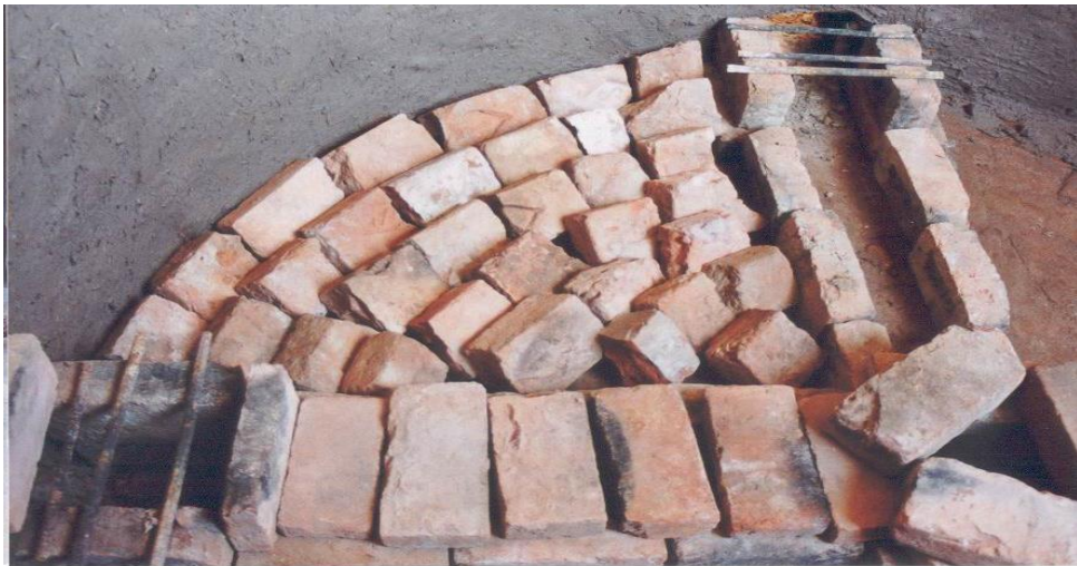
Figure 3: Arrangements of bricks on floor area of kiln; having cross and circular channel.
