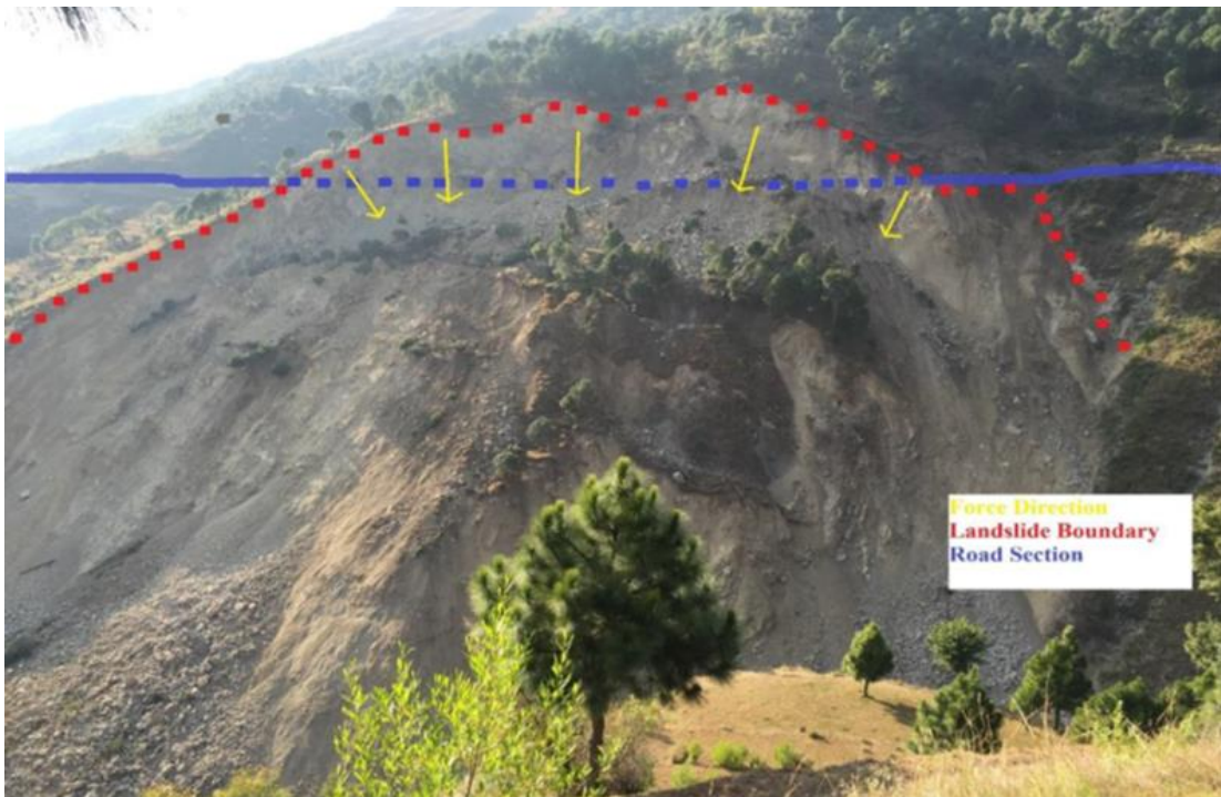
Fig- 1: Failure surface of Havelian Landslide, the collapsed section of the road is highlighted in blue.
