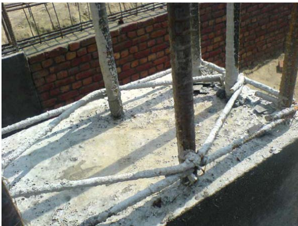
Figure-2 Another view of Hoop reinforcement with 90° bend
