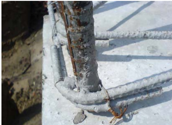
Figure-1 Hoop reinforcement with 90° bend.
