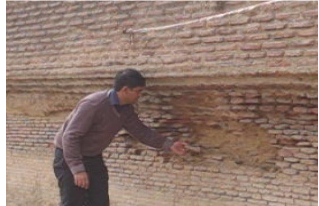
Figure 17. Visual inspection and collection of mortar sample from outer side of northern wall of Shalimar Garden
