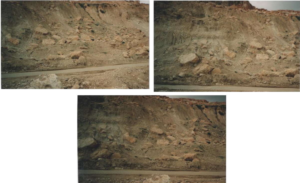
Figure 8: Circular type failures in Nammal formation
