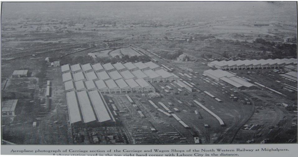
Fig. 2: Railway Workshops at Mughalpura during 1924-25
