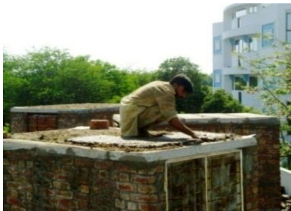
Fig. 3 Roof while Preparation
