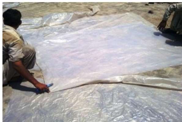
Fig. 2: Polythene sheet laying
