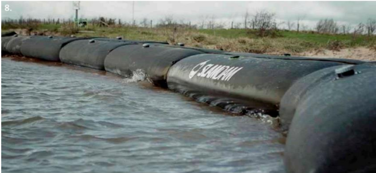
Figure 6: A Typical Rubber Dam
