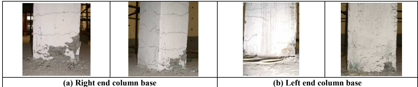
Figure 5 Damage photos at column base sections in OFT at ± 32kN lateral load
